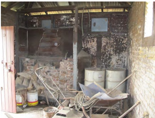
Figure 61. Interior of gent's toilet.
