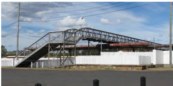
Figure 55. Western end of footbridge, near Station.
