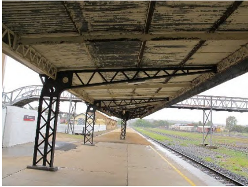
Figure 53. Cantilever type platform awning.
