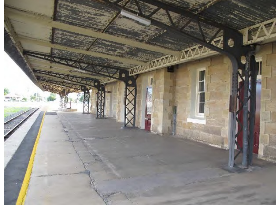
Figure 40 Railway platform on western side of station.
