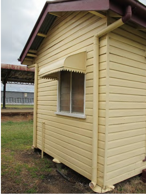
Figure 108. Exterior of ambulance room.
