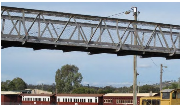
Figure 57. Footbridge over railway tracks
