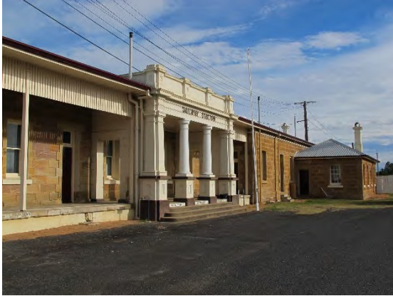
Figure 39 Eastern façade of passenger station.
