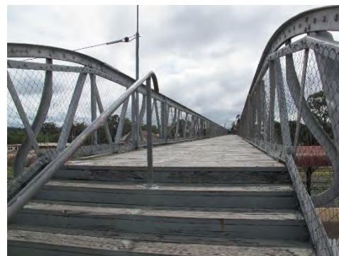
Figure 58. Timber steps and deck of footbridge.
