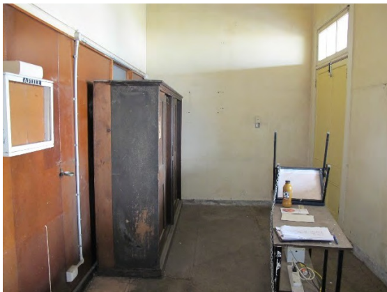
Figure 47. Former Telegraph Office divided into smaller spaces.
