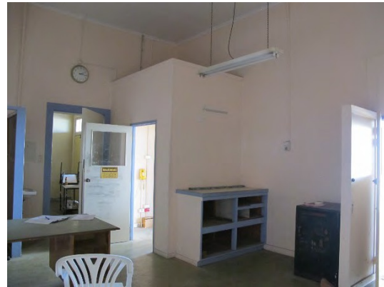
Figure 46. Inserted partition wall in Parcels Office.
