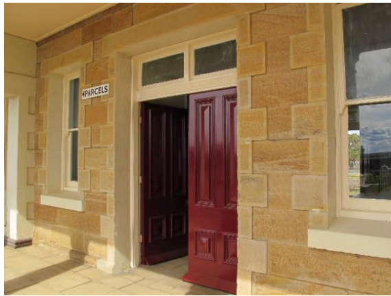
Figure 42. Sandstone walls with quoins to door and window openings.
