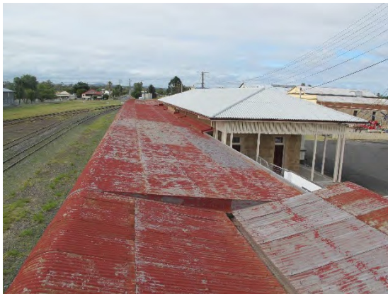
Figure 97. Top of awnings showing join between cantilever and butterfly roofs. Figure 98. Cantilevered platform awning.
