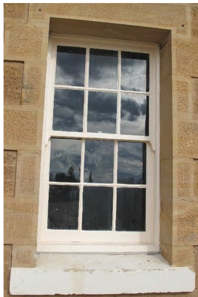
Figure 89. Six-light original window in kitchen wing.
