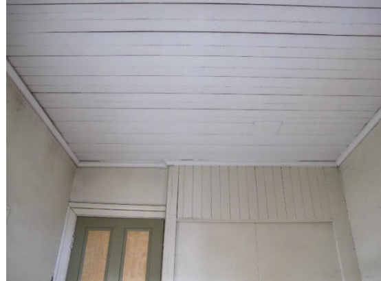
Figure 84. Original timber ceiling and plaster walls in room 12.
