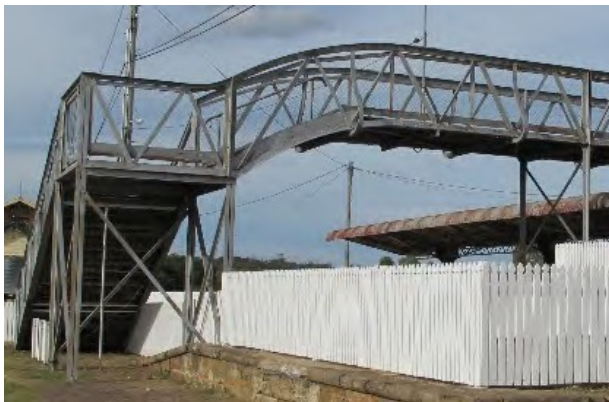
Figure 100. Steel footbridge at Lyons Street end.
