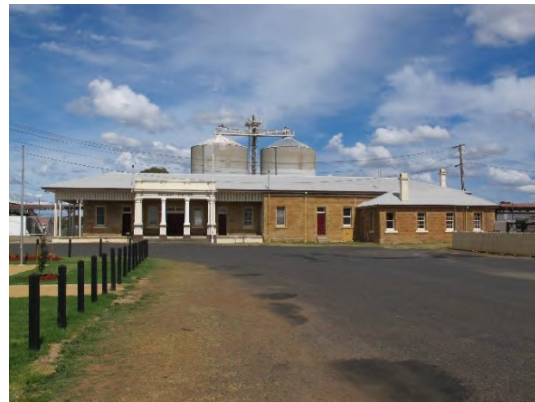
Figure 38 Eastern elevation of Warwick passenger station, kitchen wing at right.
