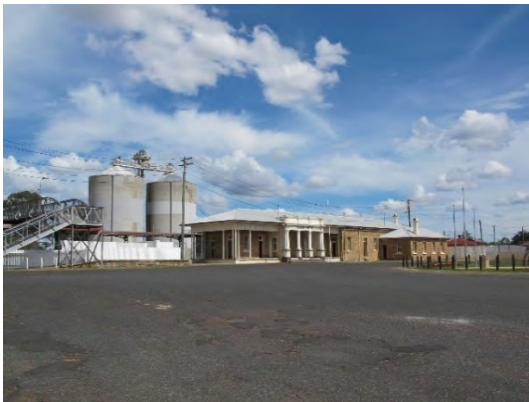
Figure 37 Forecourt of Warwick passenger station with footbridge at left and memorial park at right
