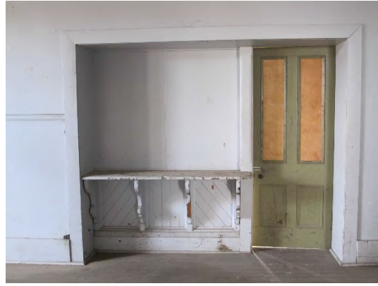
Figure 50. Original servery in former refreshment room.
