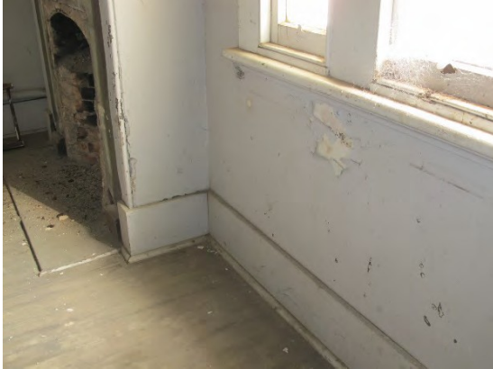
Figure 83. Original plaster wall in room 6. 12.
