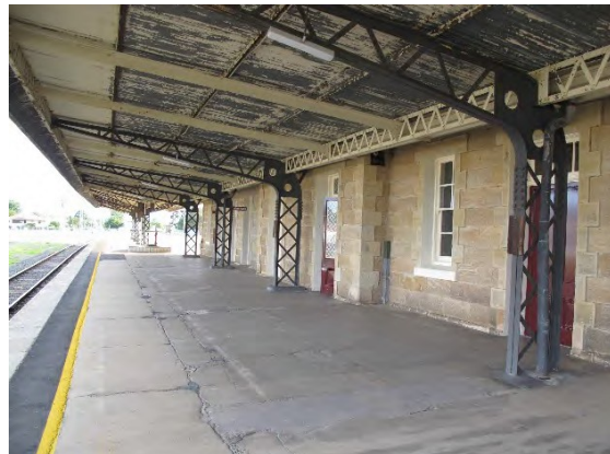
Figure 97. Top of awnings showing join between cantilever and butterfly roofs. Figure 98. Cantilevered platform awning.
