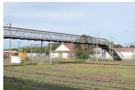
Figure 56. Eastern end of footbridge.
