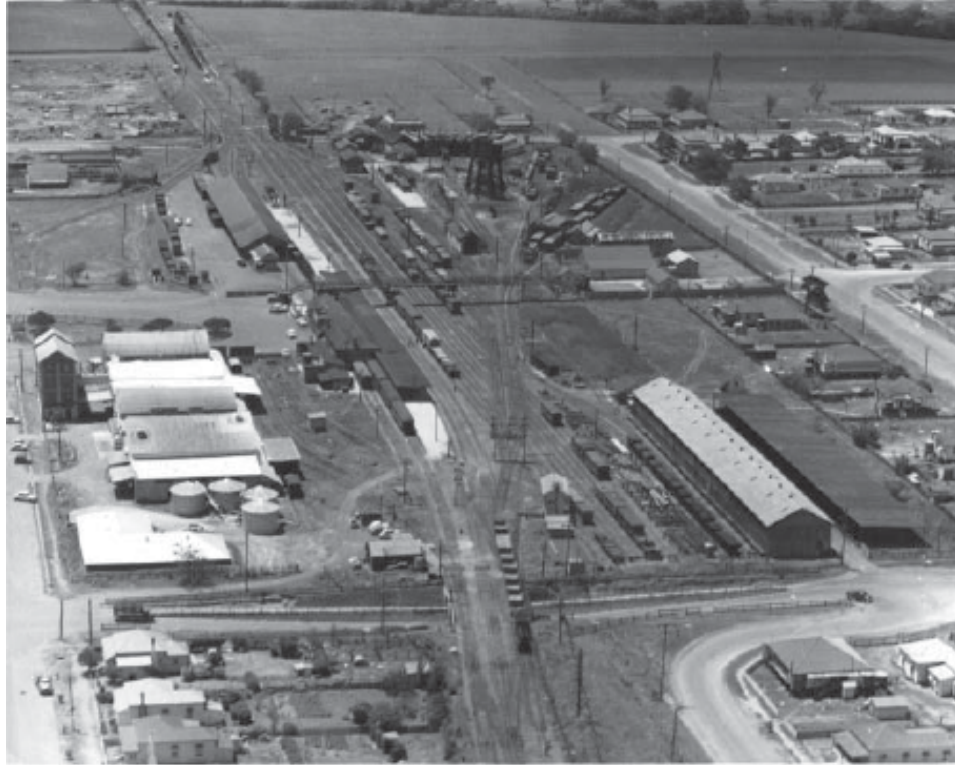
Figure 34 Warwick Railway Station Complex, 1950s, aerial view showing the two butterfly shades from 1925 at either end of the platform, and the cantilevered platform shade erected in 1936 in place. Source: Southern Downs Steam Railway - Taken from (Buchanan Architects, 2003)
