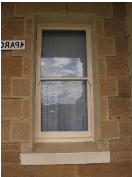
Figure 88. Single-light reproduction window in room 1.
