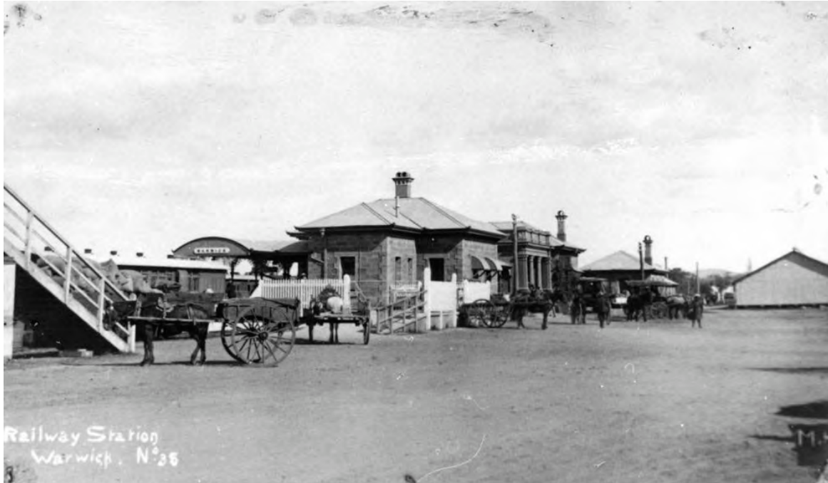
Figure 22 The Warwick Passenger Station in 1910 showing the driveway area prior to being redesigned in 1913. Source: Picture Queensland
