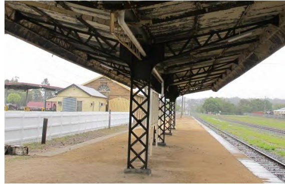
Figure 54. Butterfly type platform awning.
