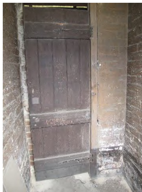
Figure 107. Original toilet cubicle with timber door.
