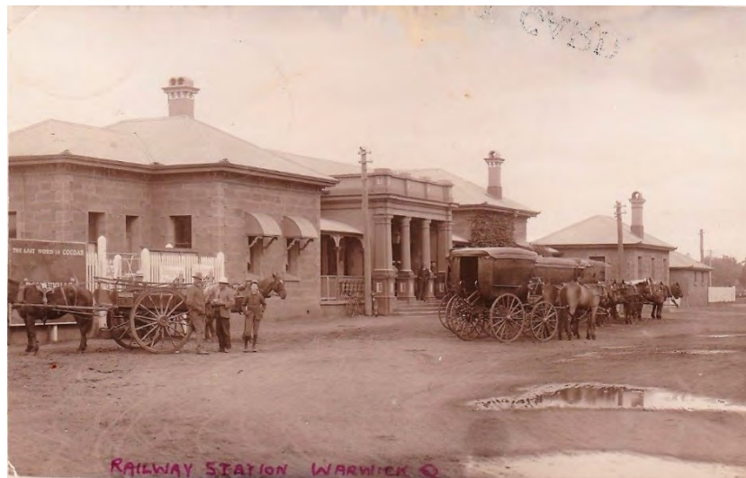
Figure 68. Photograph of Warwick railway station before the 1912 addition - note the curved verandahs each side of the portico, window hoods and single-light windows. Source: Trove
